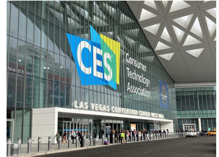
Tech East(西館)
